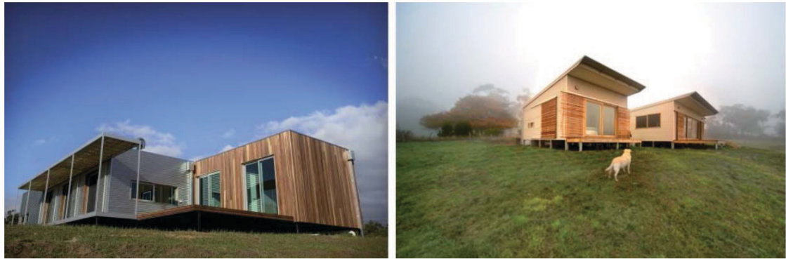
Figure 6 dan 7 Volumetric prefabricated houses (Source: Luther, 2009; Modscape®, Prebuilt®)
